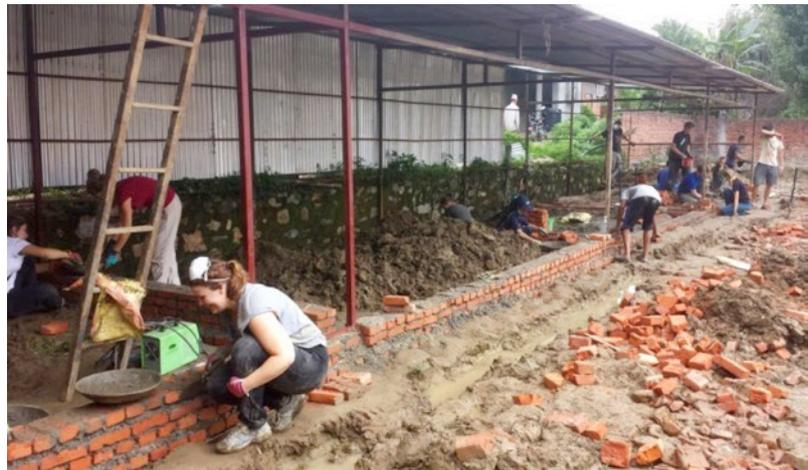
Completing the brickwork that will contain the raised 9" floors
